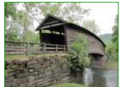
Humpback Bridge Photo by Philip deVos
